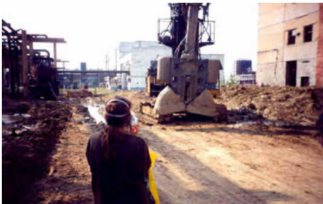
FIGURE 2. Construction of the bentonite cutoff wall.
