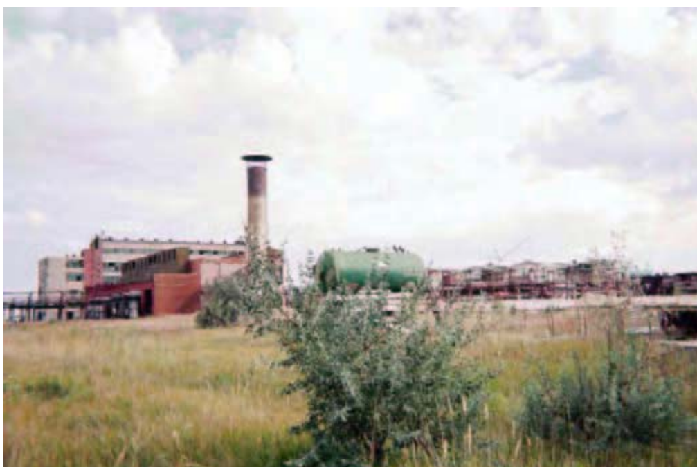
FIGURE 1. Former mercury cell chloralkali plant, Building 31.
