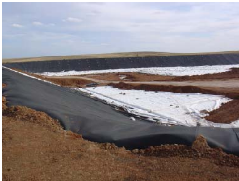
Figure 5. Containment of the landfill cell base.
