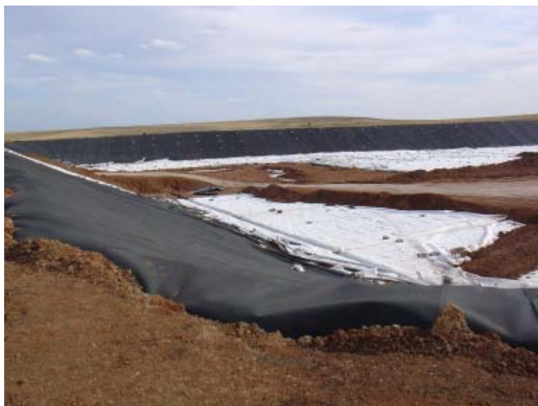
Figure 5. Containment of the landfill cell base.
