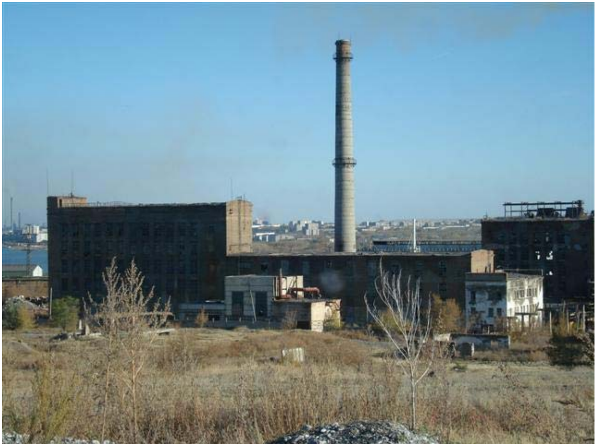
Figure 1. General view of the former acetaldehyde production factory.
