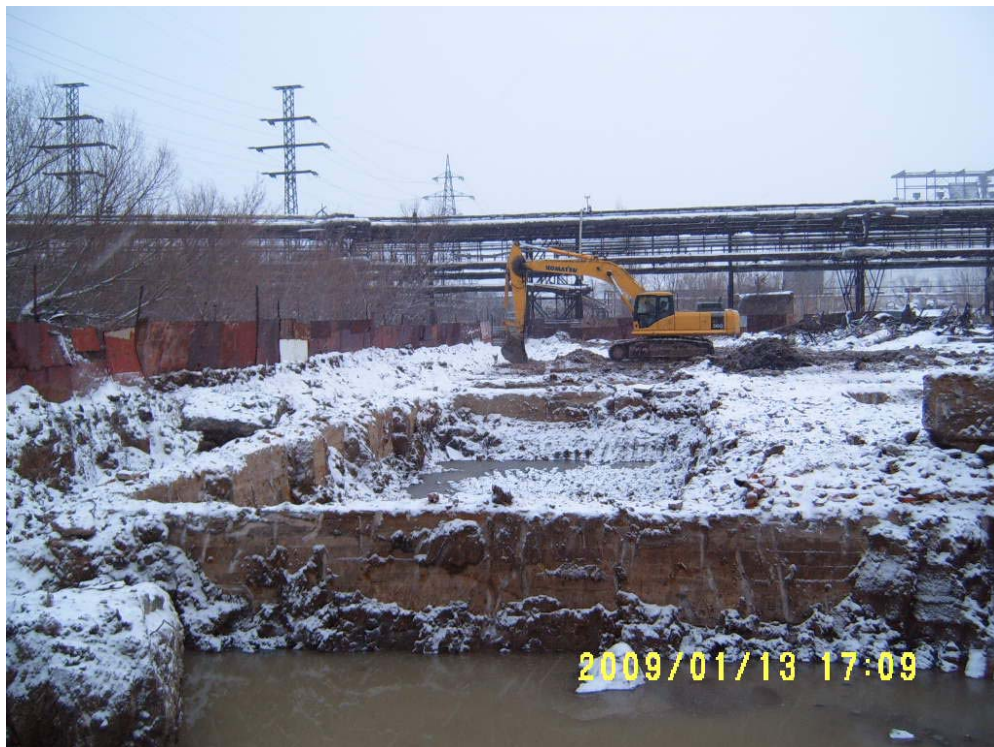
Figure 3. Excavation of soil from the base of factory buildings.
