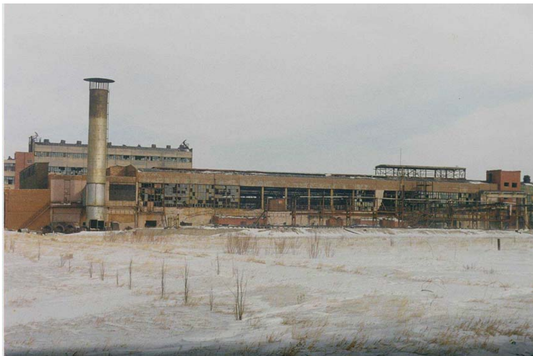
Figure 2. Electrolysis factory after closing down chlor-alkali production in 1993
