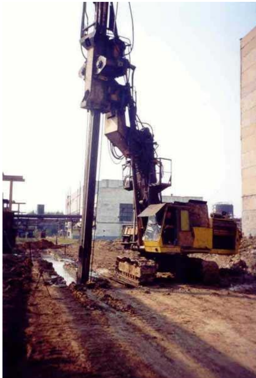
Figure 3. Construction of anti-filtration barrier “cat-off wall” around electrolysis factory
